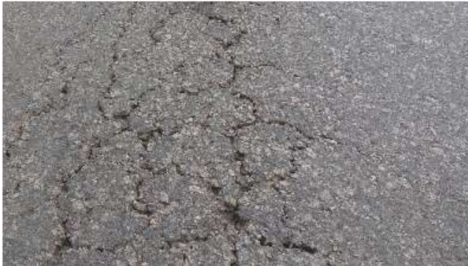
Alligator Cracks
